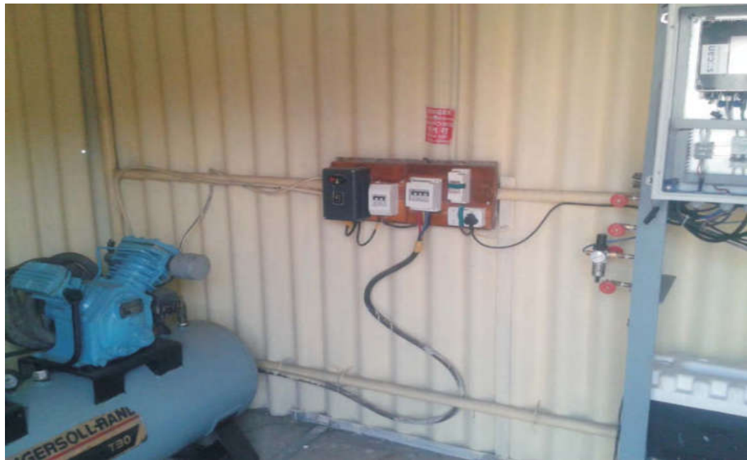
System for Treated Water Monitoring
