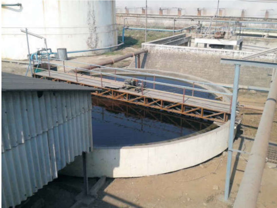
Secondary clarifier old stream
