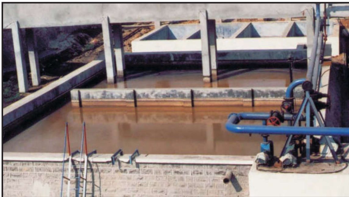
New equalization tank and feeding system to old and new stream 20 M 3 /hr.+ 70 M 3 /hr.
