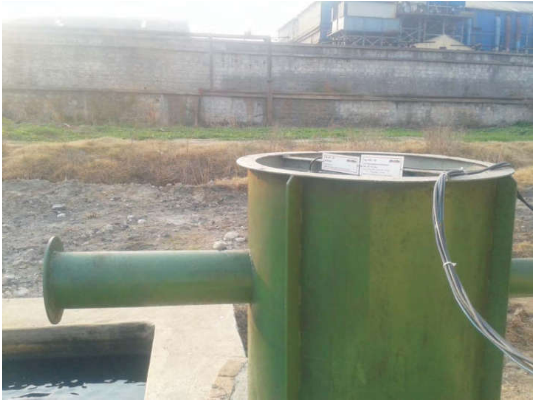
Treated Water outlet Tank
