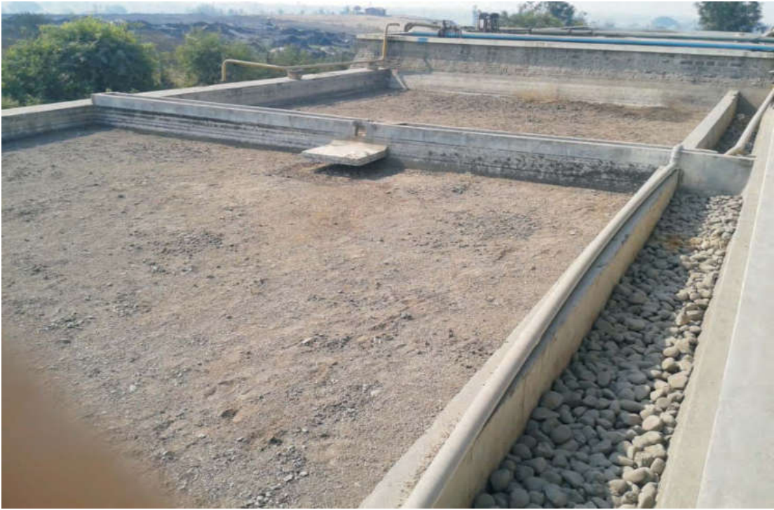
Sludge Drying Bed
