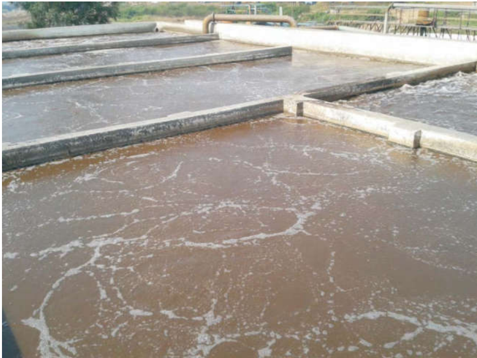
New diffuse aeration tank
