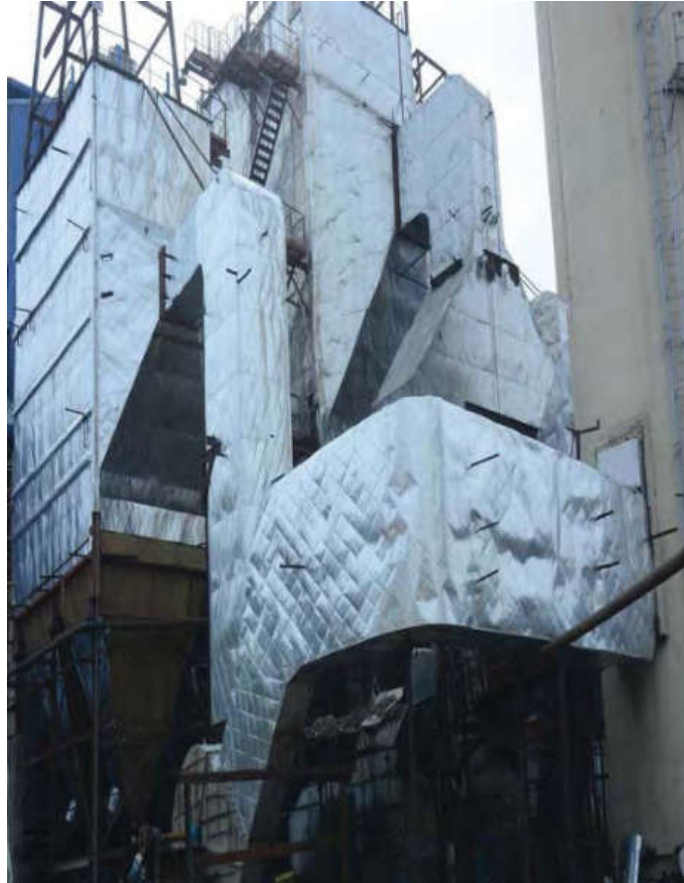
Electro Static Precipitator for 20 M.T/hr Boiler Capacity
