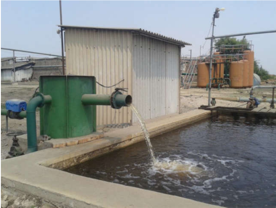
Treated Water Outlet
