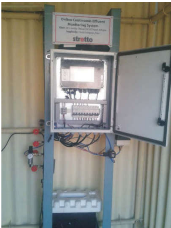
Analyzer for outlet Treated Water - for parameter pH, T.S.S, C.O.D & BOD measurement.
