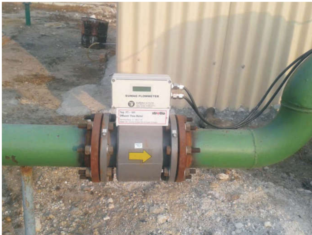
Flow meter for outlet Treated Water
