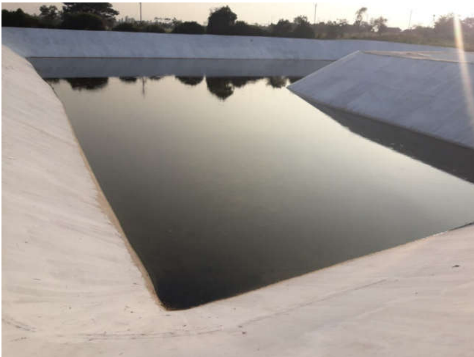
15 Days Storage Tank-2
