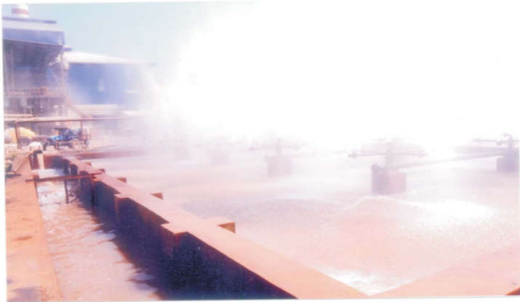
Mini spray pond capacity 10200 M 3 /day water recycle inlet temprature 58°C to 60°C outlet temprature 28 to 30°C
