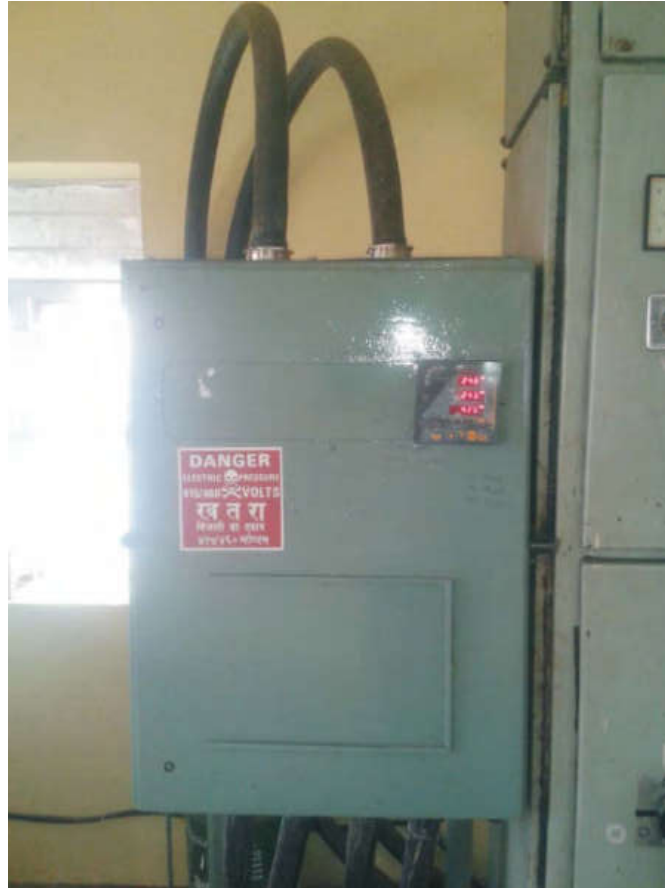
Electric energy meter for E.T.P.
