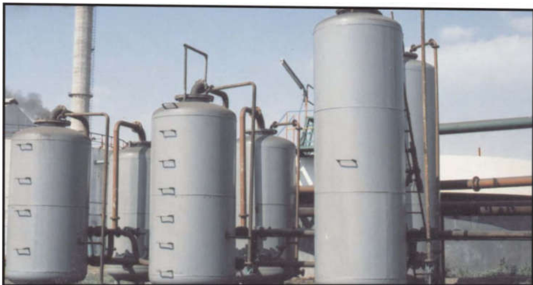
Tertiary system to streams 100 M 3 /hr. each Power sand filter followed by plant based activated carbon & polishing unit comprising high grade anthracite and activated carbon
