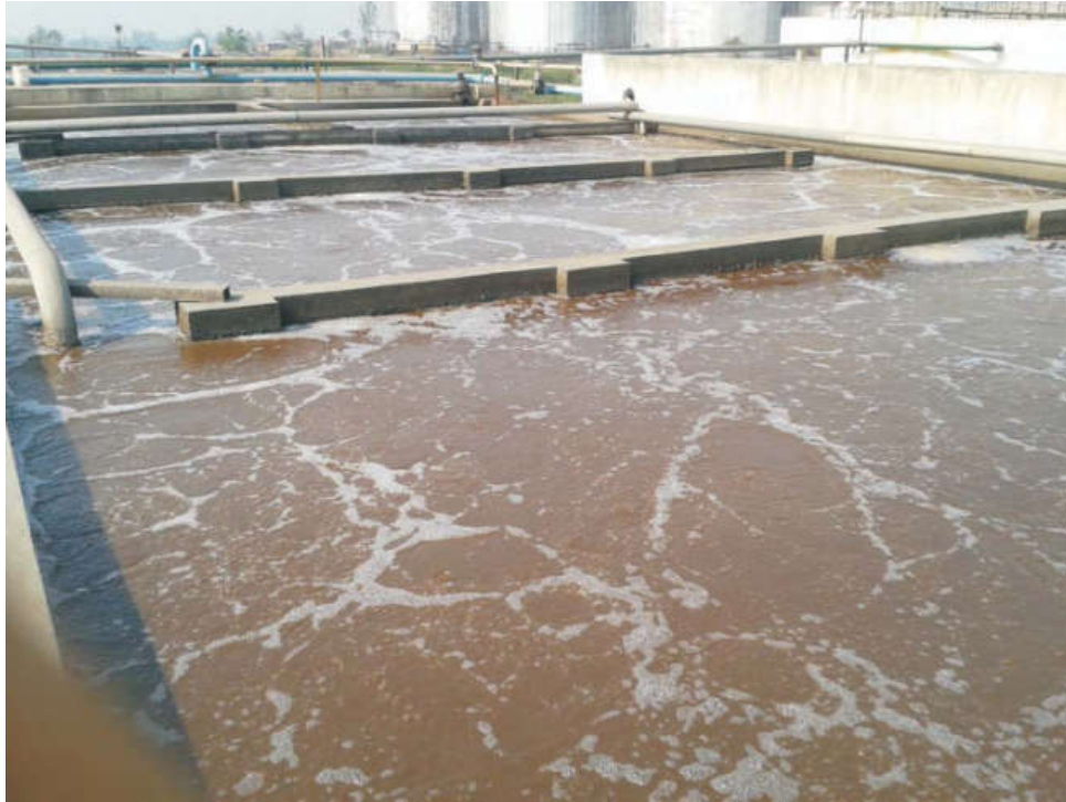
Old diffuse aeration tank
