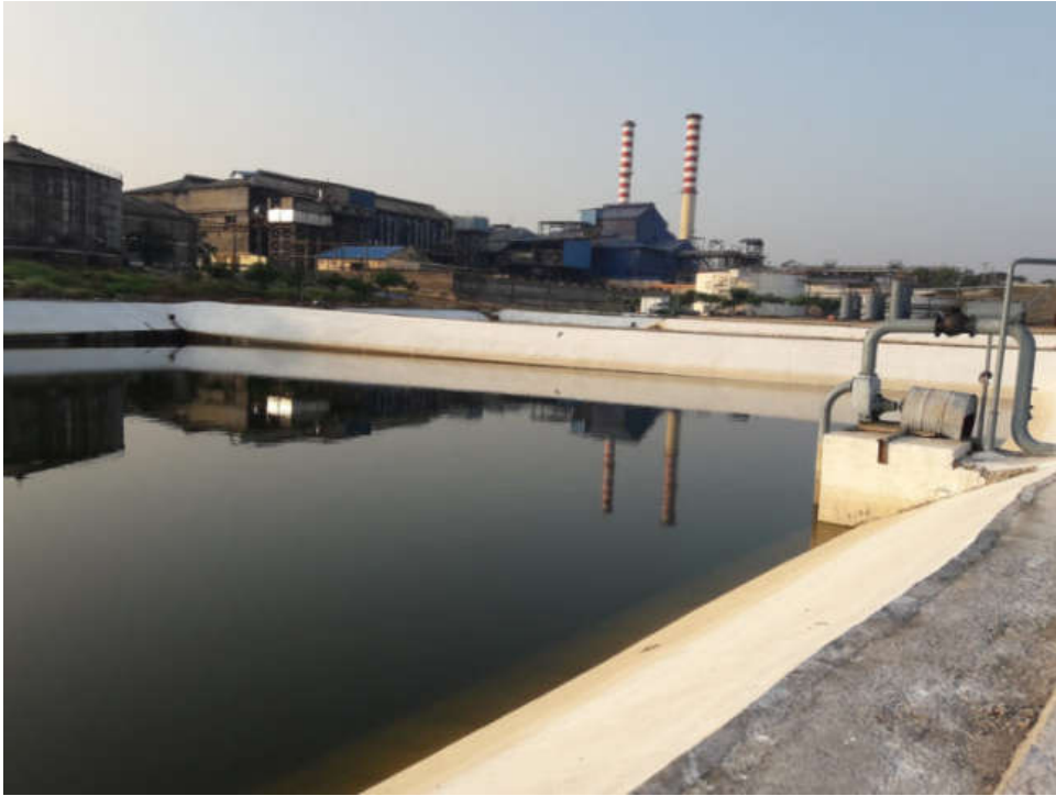
15 Days Storage Tank-1
